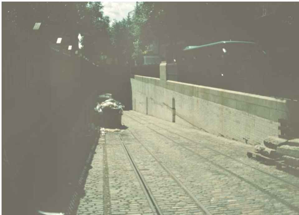
Photo 2: The last 'Cross River Tram' – north entrance to Kingsway tram Tunnel, August '08.
